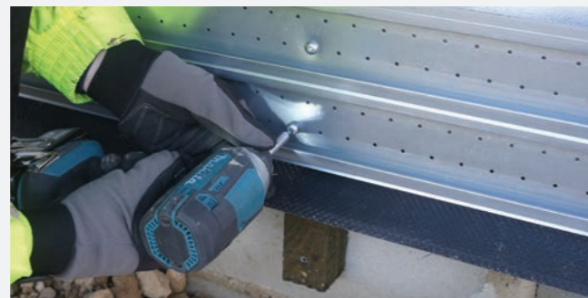
2 Interlocking rails are screwed to the structure, with fixing points at a maximum of 600mm centres.
