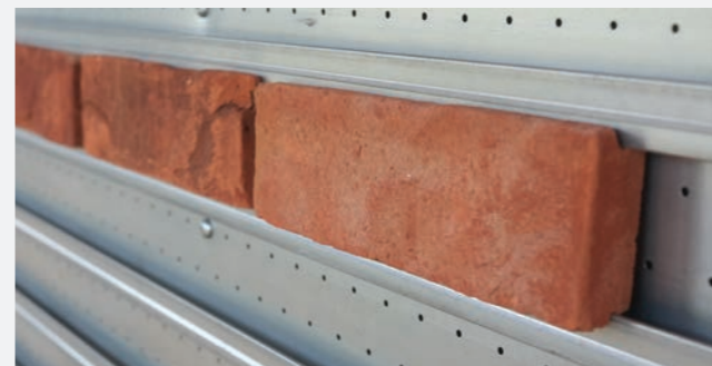
3 Specially profiled bricks are then simply clipped or slid into place before finishing with pointing mortar.
