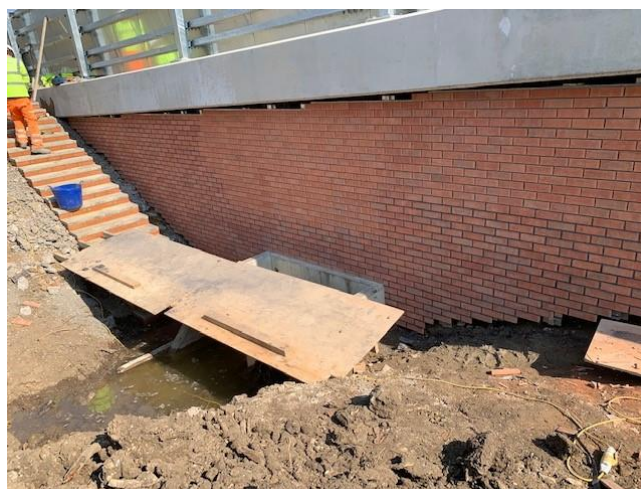
The start, the middle and the end of the wall 112 metres, 1.6 metre high 150 Square metres
